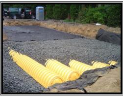
N&P/NP&V prepared site development plans for park and shoreline improvements for the Village of Poquott. A stormwater management system using a variety of shallow sub-surface systems and a bio-retention area was designed to address significant runoff from upland areas into the Harbor. Additionally, a shoreline restoration/bank stabilization plan was prepared to address shoreline erosion and the existing boat ramp was re-constructed/expanded to improve access.
